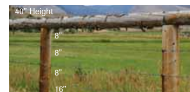
Pressure-treated poles are recommended. Top rail 4" diameter and 13' long. Posts 5"-6" diameter and 8' long. Posts set on 12' centers.
